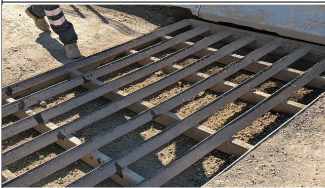
Site Access Road to Adams Road – rumble grid.
