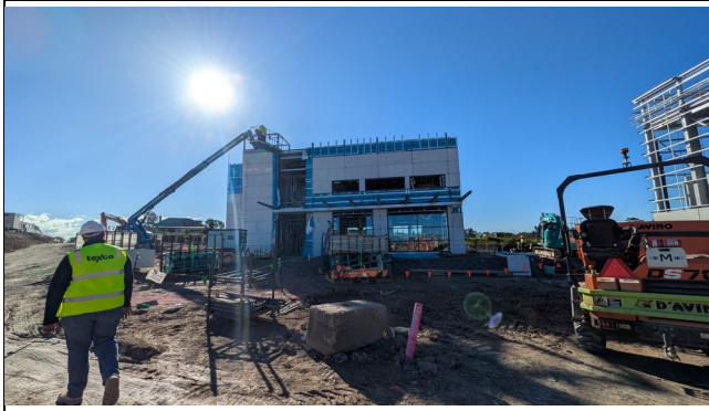
Administration building construction with some glazing installed.
