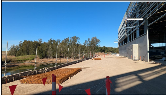
Eastern boundary retaining wall constructed.
