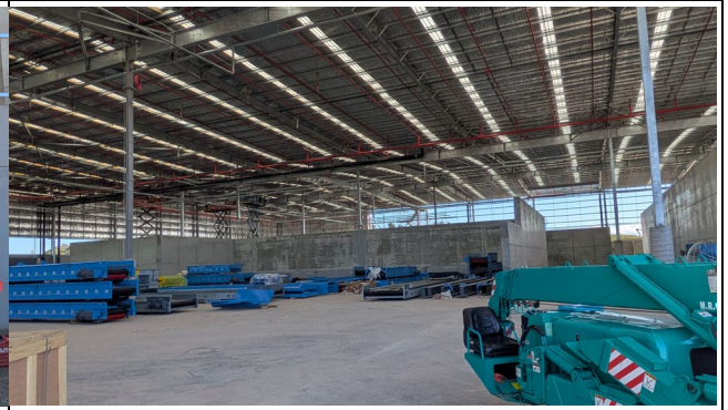
Warehouse interior with slab, structure & roof complete.
