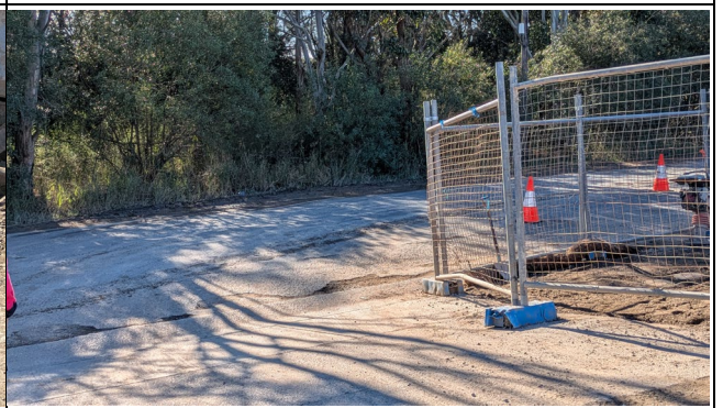
Site Access Road to Adams Rd – no appreciable tracking.
