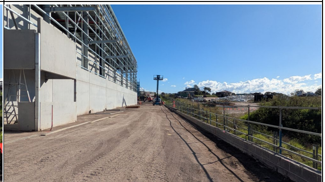
Northeastern and eastern retaining wall and stormwater works ensure site is self-contained.
