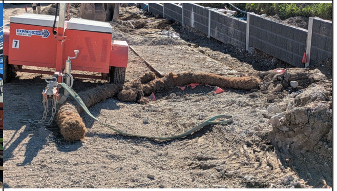
Northern half of access to Adams Rd installation of utilities near completion – ErSed controls in place.
