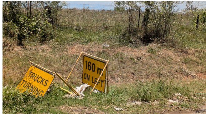
Traffic control signage on Adams Road in accordance with CTMP.
