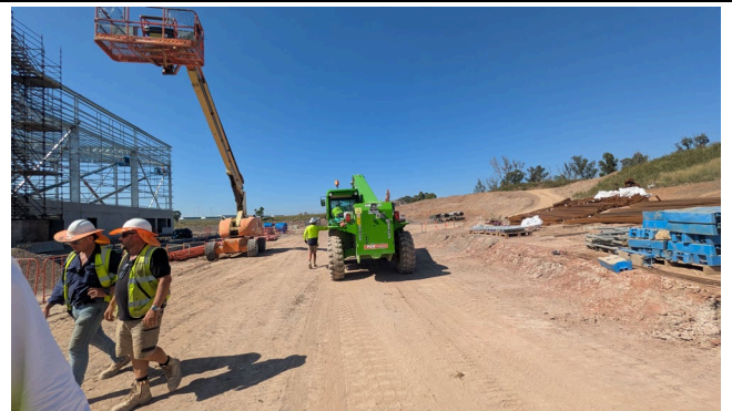
EWPs operated for steel installation use non-tonal alarms.
