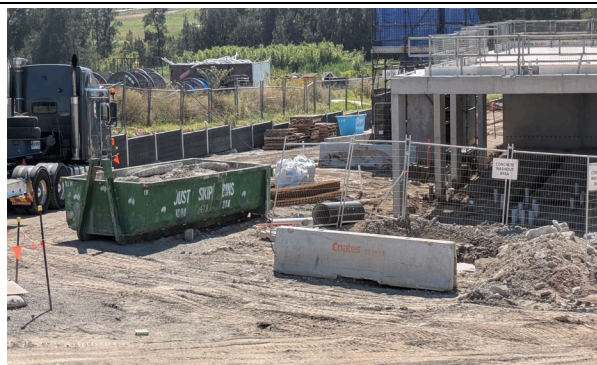
Concrete washout is well implemented and neat.
