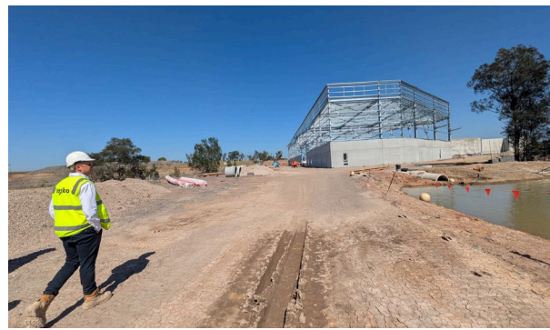
View west of the southern boundary showing steel structure installation.
