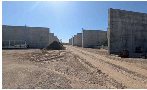
Warehouse push walls and bay walls.
