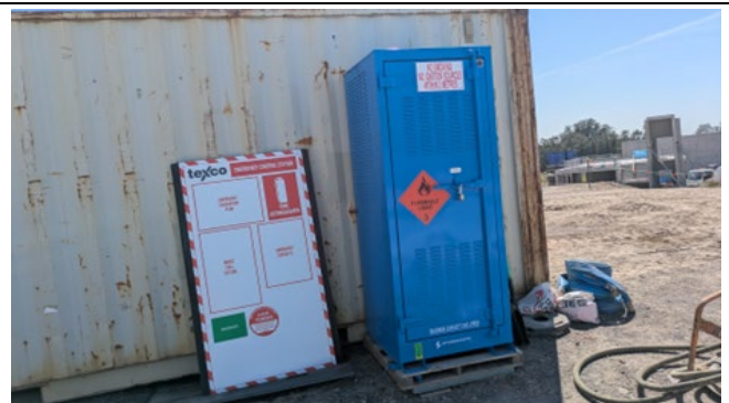
Dangerous goods stored in robust bunded dedicated stores.
