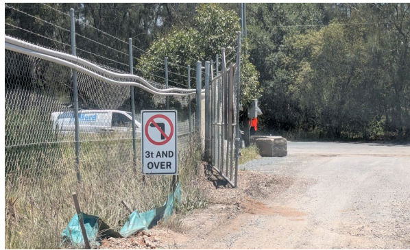
Site access signage restricts access by 3 tonne and over vehicles to Northern Rd in accordance with CTMP.
