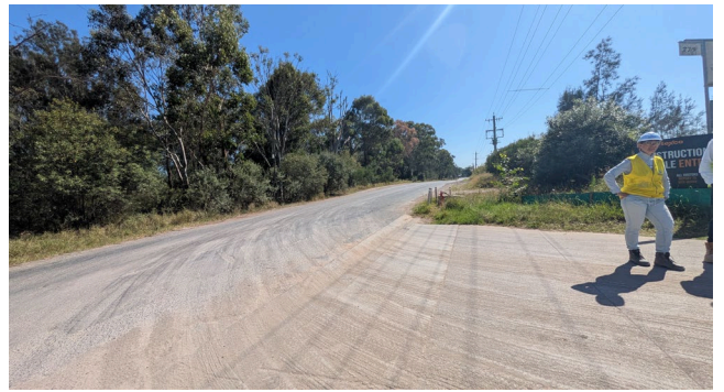
Site Access Road to Adams Road – no appreciable tracking.
