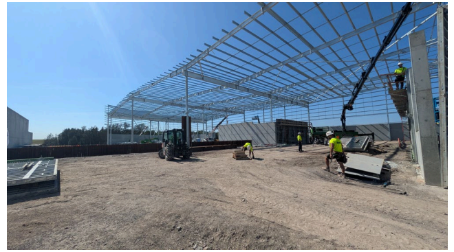
Structural Steel Installation.
