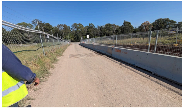
Site Access Road to Adams Road – rumble grid.
