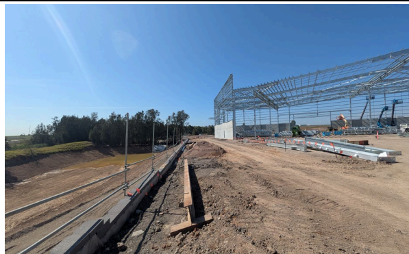
Eastern boundary retaining wall constructed.
